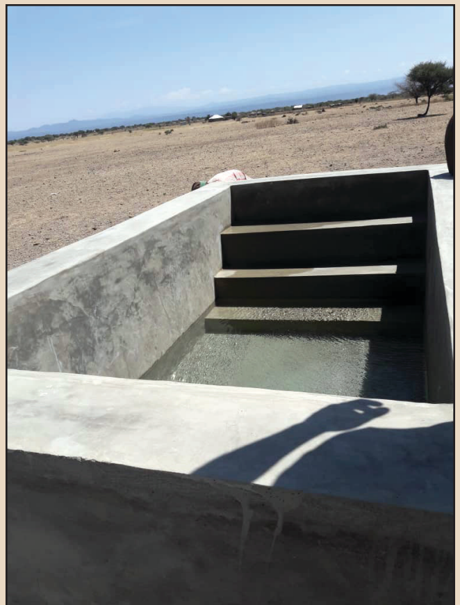
Baptismal being filled with water after repairs completed
