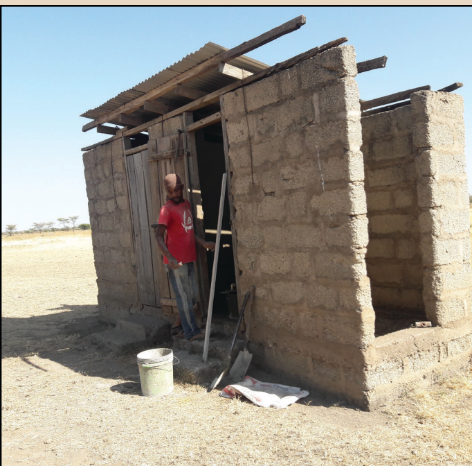
Repairman working on Church bathroom
