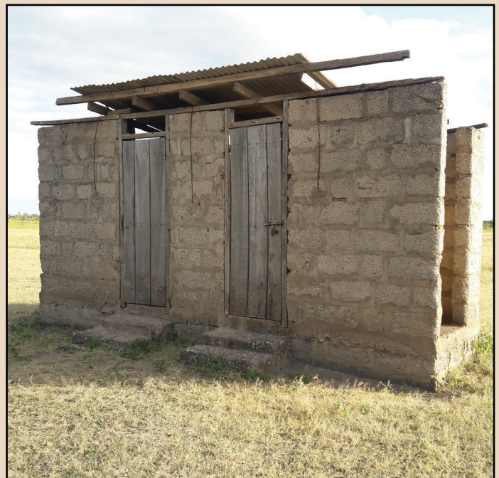
Church Bathroom repairs completed
