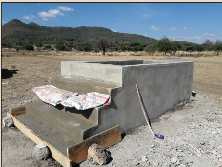
Repair work underway on existing baptismal with addition of cement steps
