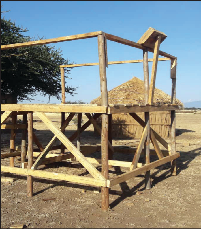
Construction of outdoor crusade stand for Maasai church nearly completed
