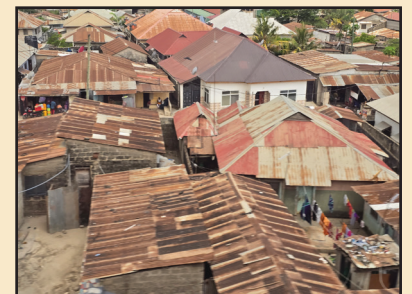
View of rusted tin roofs in Dar es Salaam Tanzania from the elevated train platform
